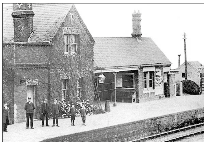
Old North Road Station at Longstowe Photo from John Mann collection
